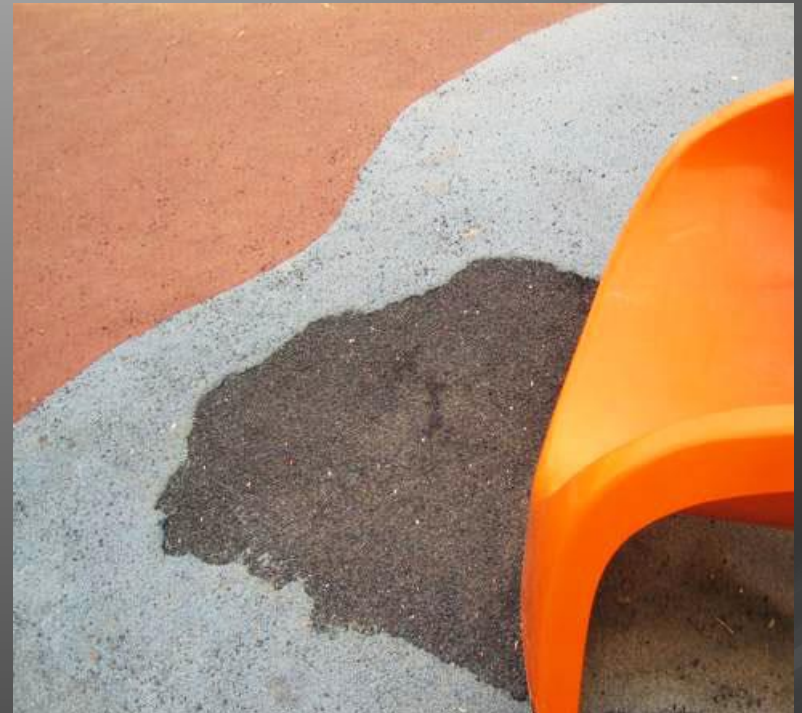
Destruction of the EPDM surface in problem areas (e.g. under slides or swings)
