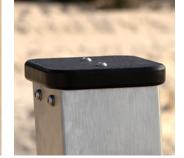
Safe end caps on top of the structure made of synthetic material,
